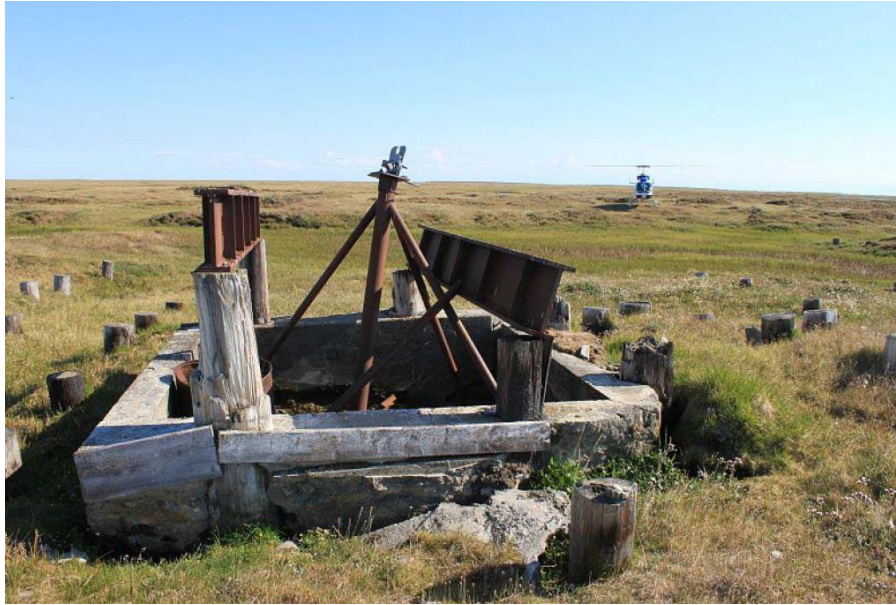
Figure TM5-9. View of South Barrow #3 well. The well has a concrete cellar and steel beams stacked on pilings that were cemented into the cellar. The well is cut off at ground level inside the cellar (BLM 2013a).
