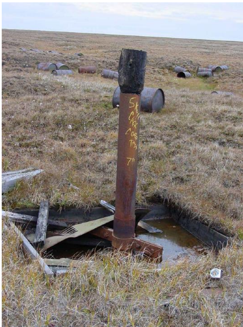
Figure TM5-10. Skull Cliff Core Test #1 and cellar. Note wooden plug at top of well casing and drums scattered around the site.
