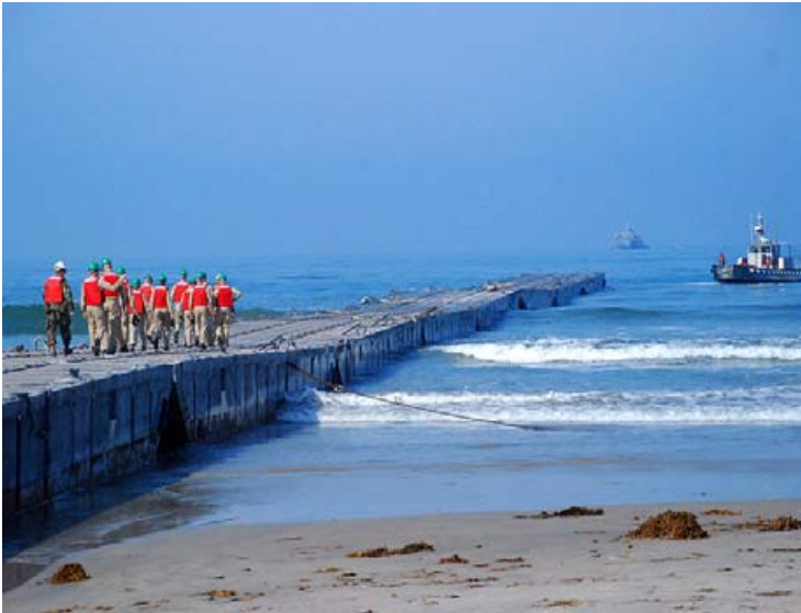
Figure 6.3-1. U.S. Navy Floating Causeway Constructed by Attaching Non-Powered Lighterage Together
