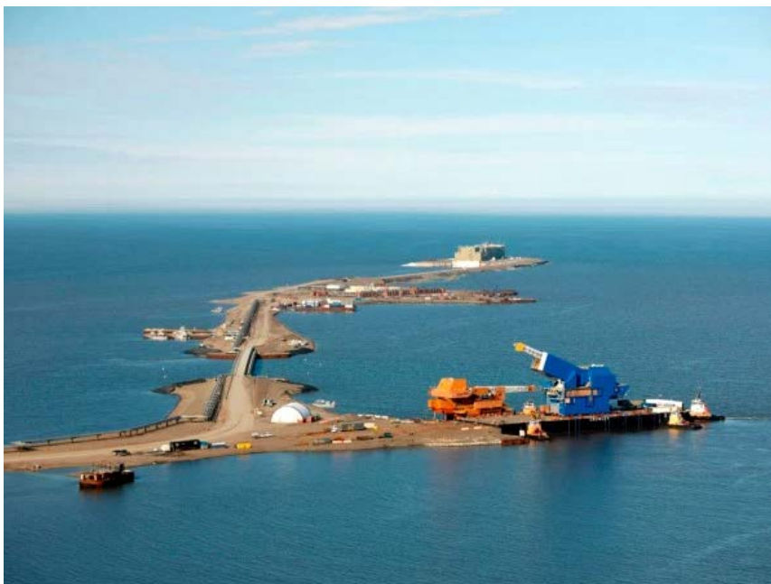
Figure 4.1-2. Parker Drill Rig Offloading at West Dock 2, Prudhoe Bay
