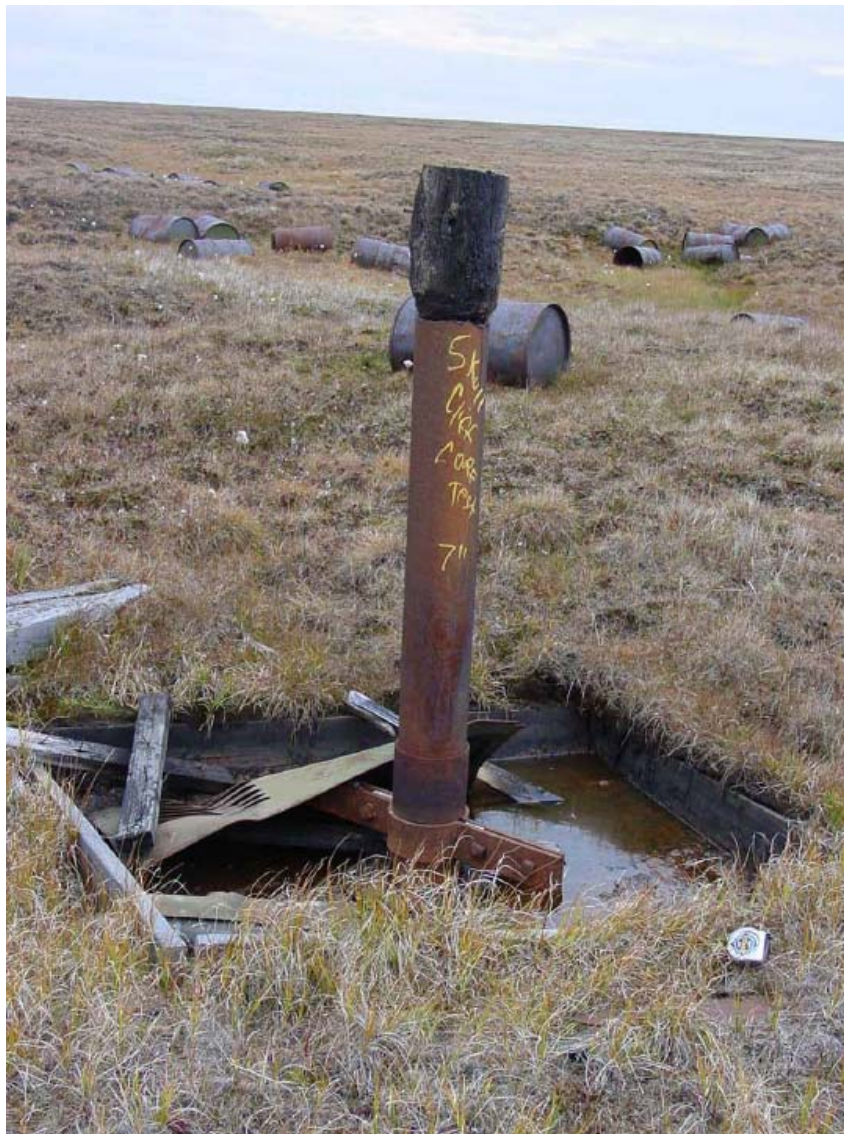
Figure TM4-4. Skull Cliff Core Test #1 and cellar. Note wooden plug at top of well casing and drums scattered around the site.
