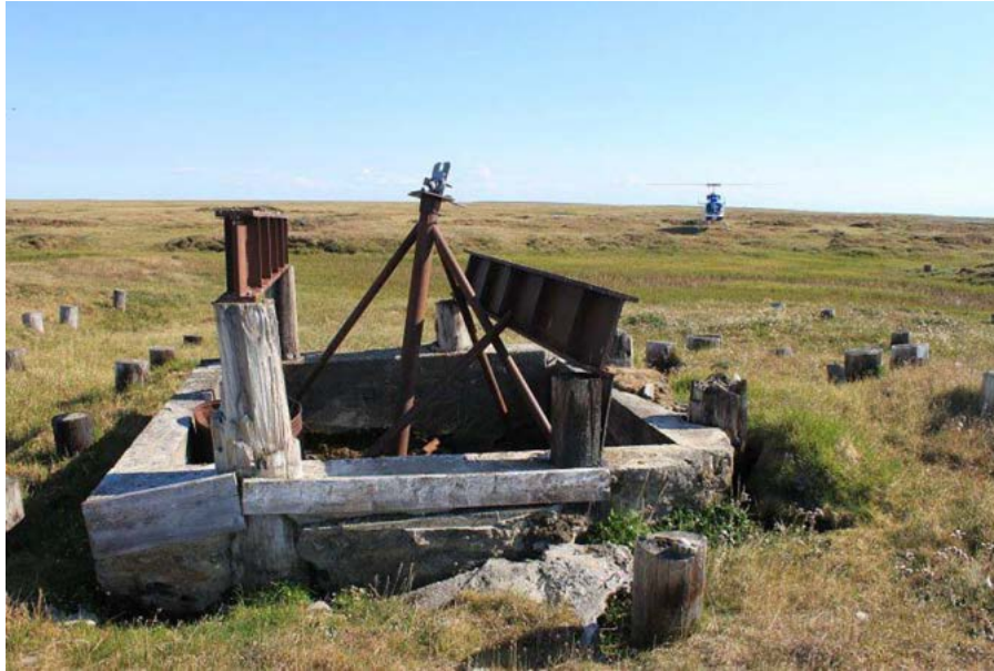
Figure TM4-3. South Barrow #3 has a concrete cellar and steel beams stacked on pilings that were cemented into the cellar. The well is cut off at ground level inside the cellar (BLM 2013a).
