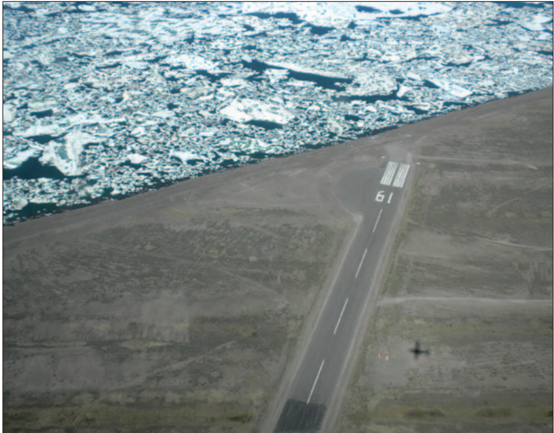
Airstrip vulnerable to erosion and flooding.
